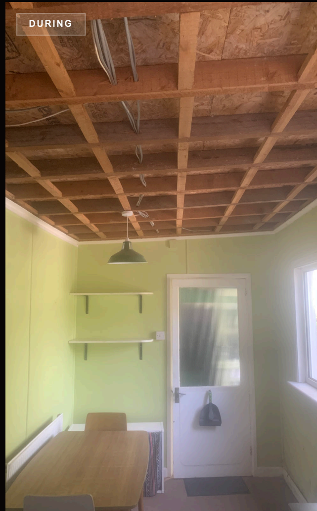
CEILING STRIPPED TO TIMBER JOISTS
